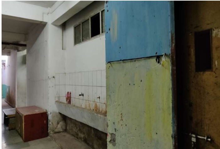
Un hygienic Toilet location
